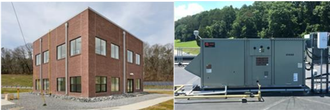
Figure E1 Two-story Flexible Research Platform (left) and RTU on the FRP (right) at Oak Ridge National Laboratory
